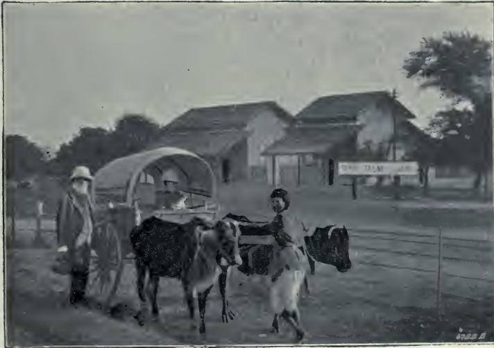
TALNI RAILWAY STATION.
